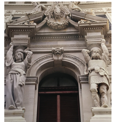
Calder’s sculptures North façade
